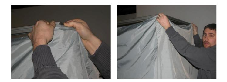
13. Using rubber mallet tap corded fabric into the 4 corners first. This locks corners into position for the remainder of the top carriage installation.
