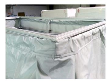
14. After the corners are secured, tap corded fabric into grooves at the center point of each side. Then tap the midpoints of each section created. Repeat this multiple times until fabric is completely secured in the groove around the perimeter. (Not following this process will create an excess fabric bundle at the corner, see bottom photo)
